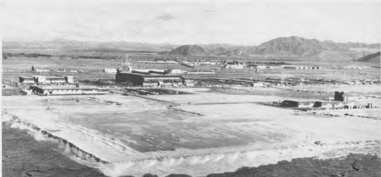
THE NAVY HAS SPENT $37,000,000 ON NAMTC AND EVENTUALLY THE INSTALLATION WILL HAVE A VALUE OF $75,000,000
