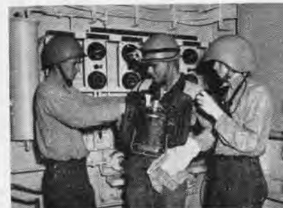
DAMAGE CONTROL PARTIES MAN STATIONS
