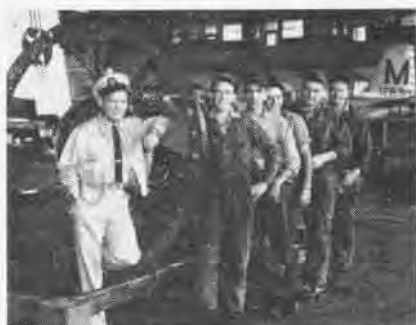
CREW WITH RECENTLY PULLED JET ENGINE
