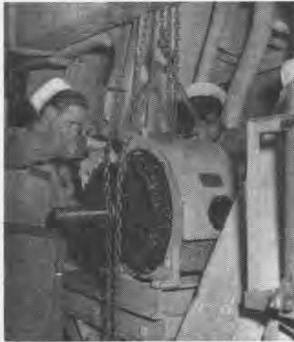
CLEANING DC-MG SET IN ENGINE ROOM
