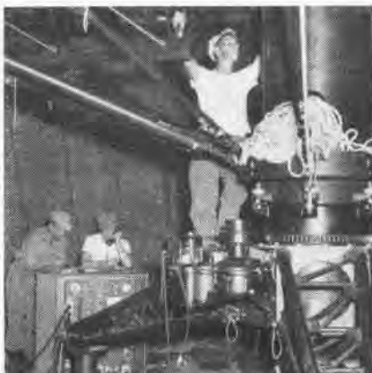
TECHNICIANS AT WORK IN NEW RADOME
