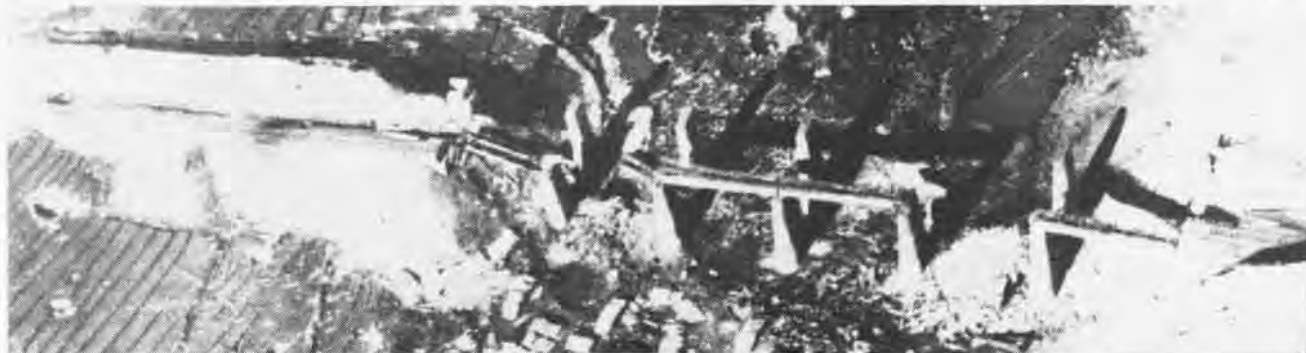
LEGENDARY BATTLE of Carlson's Canyon resulted in leveling of all new construction at spans shown above. Strikes formed background for motion picture, "The Bridges of Toko-ri." Other Korean incidents are detailed in new book, "Sea War in Korea," by Cdrs. Cagle, Manson.
