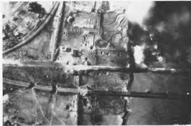
SINUJU BRIDGE crossing on the Yalu River was target of attacks and subject of squadron songs. Such attacks are included in new history.
