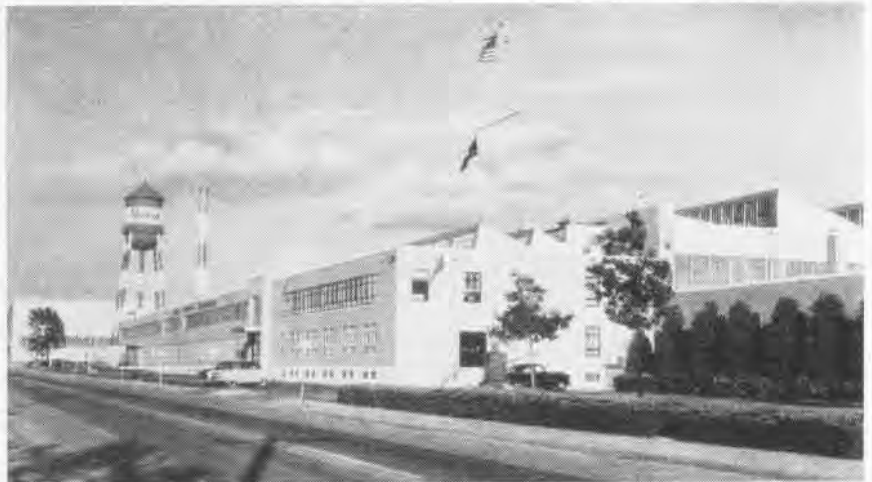
BEECH PLANT I IN WICHITA, KANSAS, GREW FROM ORIGINAL 30-FOOT-SQUARE SHOP
