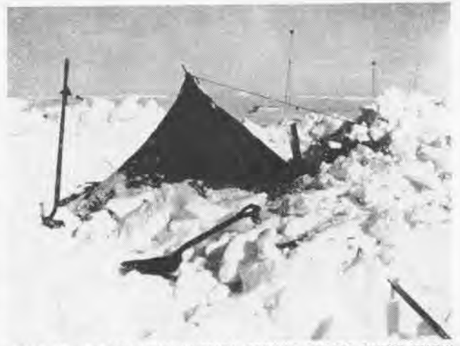
WEATHER HUT AT LITTLE AMERICA BECAME BURIED UNDER SNOW
