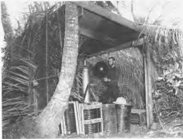
HYDROGEN GENERATOR SHELTER IS MANNED ON PACIFIC ISLAND
