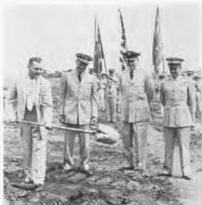
BULLDOZERS were already at work as three CO's witness ground-breaking for Atlanta.
