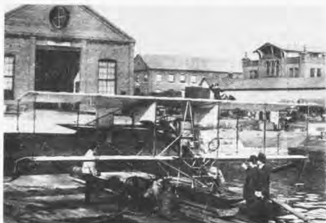
THIS CURTISS PUSHER plane was used to demonstrate the newly developed compressed air catapult at the Washington, D. C. Navy Yard.
