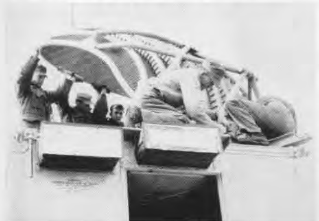
SIX HOURS after landing complicated GCA equipment was in operation and Norwegian Air Force pilots were making practice runs.
