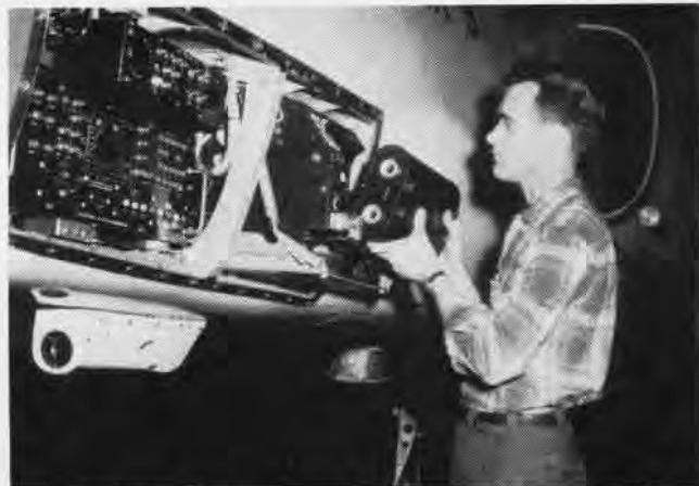
OSCILLOGRAPH MAGAZINE TAPES OUTPUT OF ELECTRICAL SYSTEM
