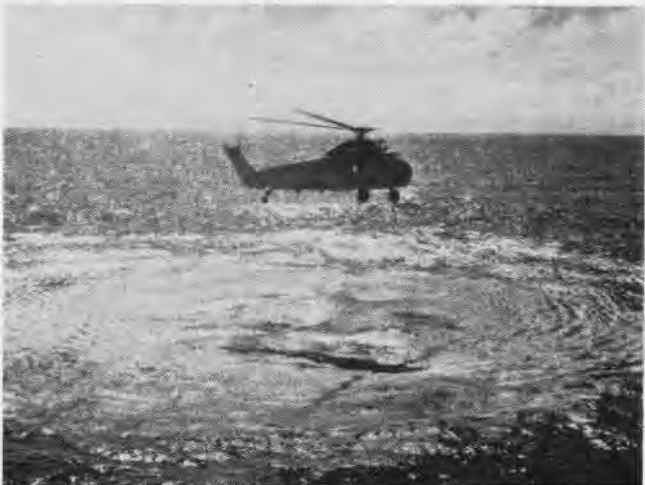
HOVERING OVER CONTACT, H5-7 COPTER LOWERS ITS DIP SONAR
