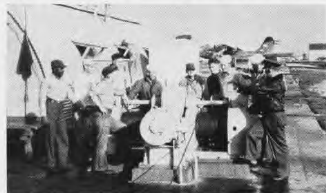
CHIEF R. H. McCROREY, (R), INSTRUCTS MEN IN USE OF WINCH
