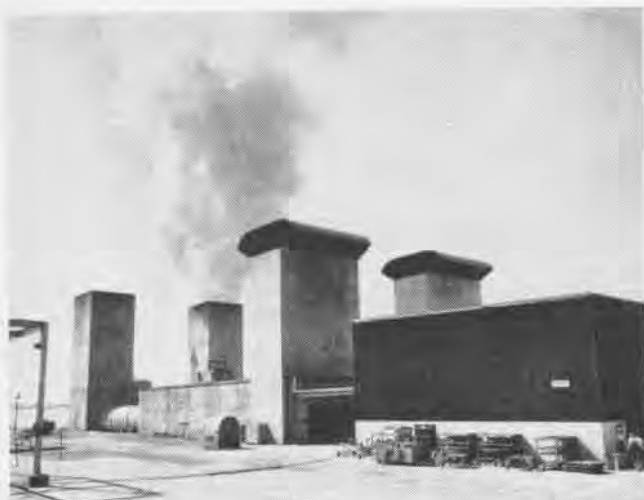
EQUIPMENT IS modern, complete—and large. This test cell at North Island provides O&R with means to test jet engines after overhaul.
