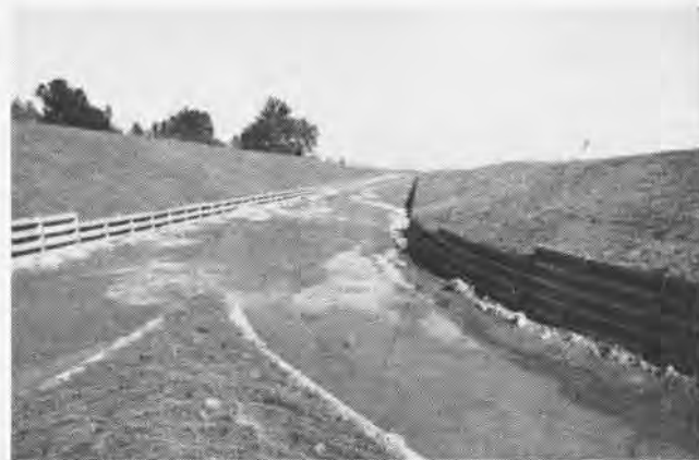
"AFTER" VIEW of same area shows startling effectiveness of soil management planning and execution. State soil experts assisted Navy.
