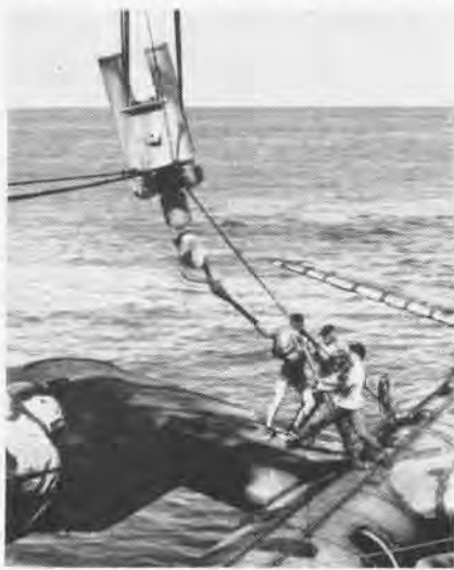
CRANE HOOK SECURED TO HOISTING SLING
