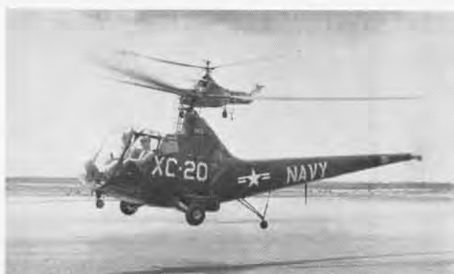
VOUGHT-SIKORSKY'S R-6A/HOS-1 was advanced version of R-4. Built by Nash-Kelvinator, had 235 hp, all metal airframe, weighed 2600 lbs.
