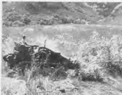
CATERPILLAR OPERATOR BEGINS CLEARING
