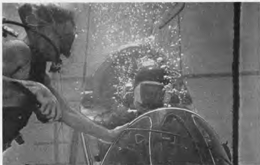
SCUBA-EQUIPPED ENGINEER observes pilot's escape technique in underwater test conducted at Air Crew Equipment Laboratory, Philadelphia. Early tests have shown that use of right method will permit pilot to trim up to 15 seconds from his escape time; since aircraft may sink up to 150 feet in 15 seconds, the faster the escape, the better the chance of survival. Other tests also were conducted in the nose down, tail down and inverted positions.
