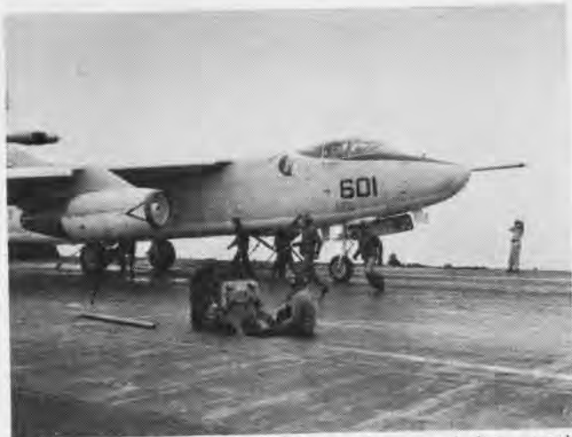
AN A-3B SKYWARRIOR straddles #3 catapult as one of three catapult crews makes final check to guarantee the aircraft a smooth launch.
