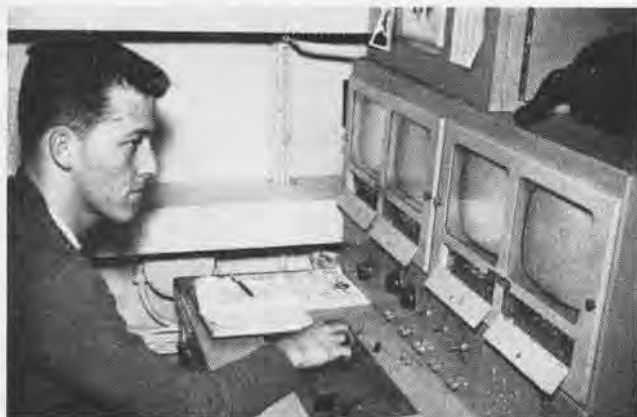
THE REMOTE CONTROL console of PLAT system installed in Independence is operated by A. L. Bender, AN. He selects best camera view.
