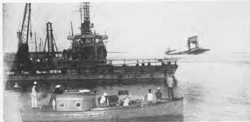
THIS PHOTOGRAPH shows one of the first catapult takeoffs made at Pensacola. The pilot of the airplane being launched off barge is Lt. Kenneth Whiting for whom Whiting Field is named.
