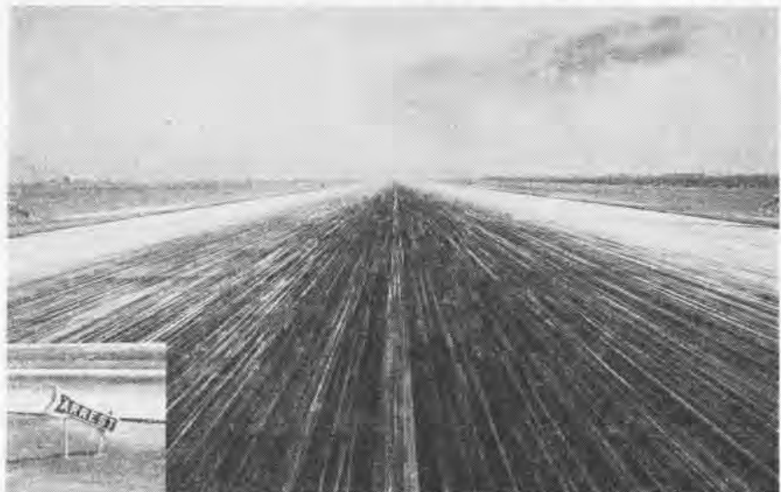
ARRESTING GEAR ARROWS at NAS Lemoore are believed by station officials to be a unique method of pointing out to pilots location of arresting gear. The arrows, internally lighted at night, are located on either side of the doorway with the word "Arrest" on each side.
