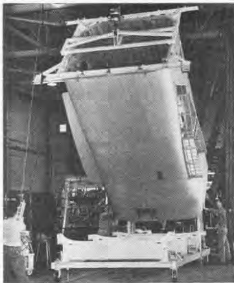
FUSELAGE was built in three sections by using vertical rigs for easy accessibility during assembly.
