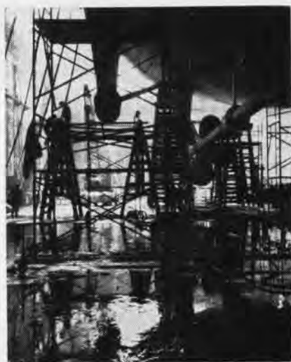
TAKEN FROM drydock floor, photo depicts yard workers replacing Forrestal's screw.
