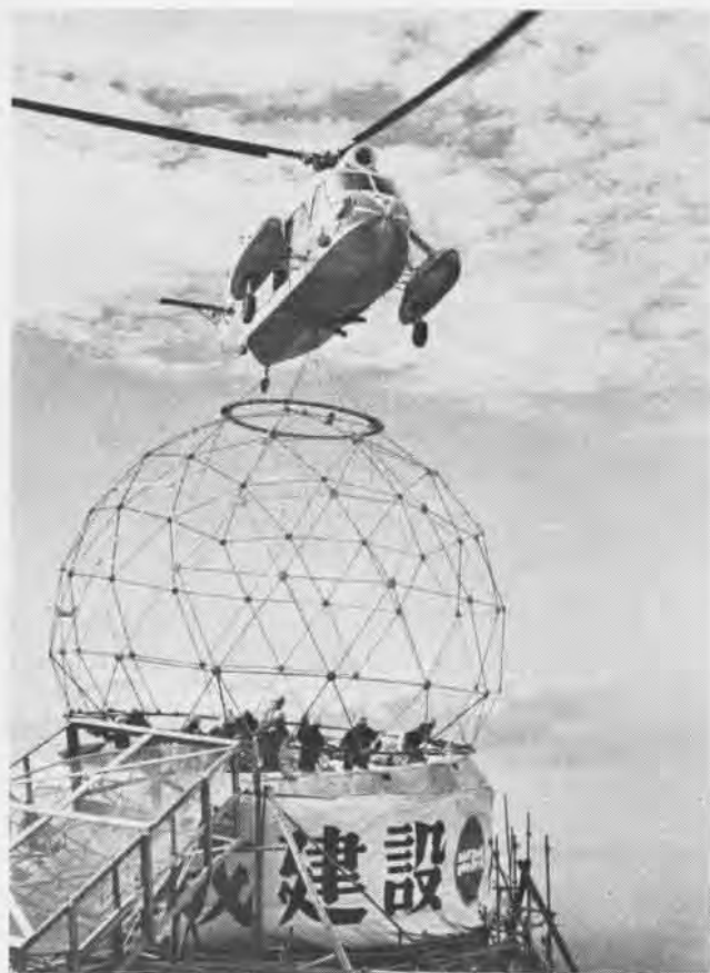
HELICOPTER PLACES RADOME ON MT. FUJI WEATHER RADAR SITE
