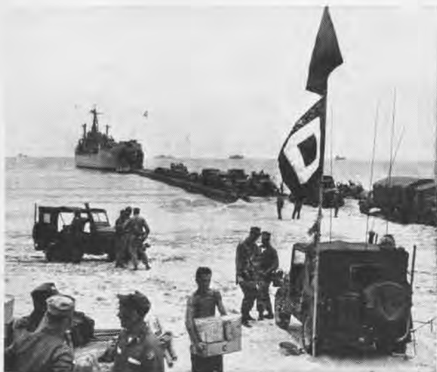
CAUSEWAY STRETCHES from LST to Chu Lai beach as vehicles come ashore to support combined Seabee-Marine airfield project.
