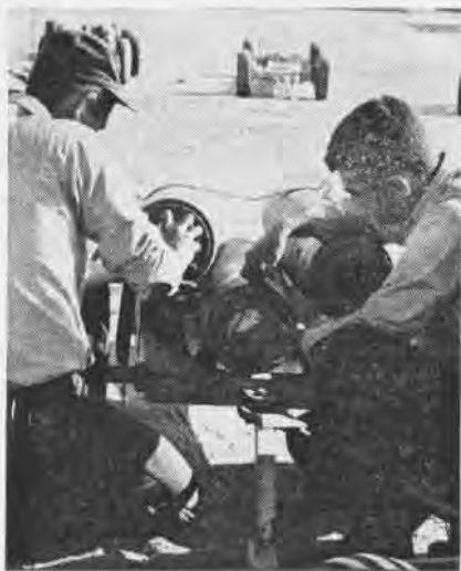
SETTING FUZES of these Snakeye bombs are D. G. Murphy and R. T. LePage, AO's.
