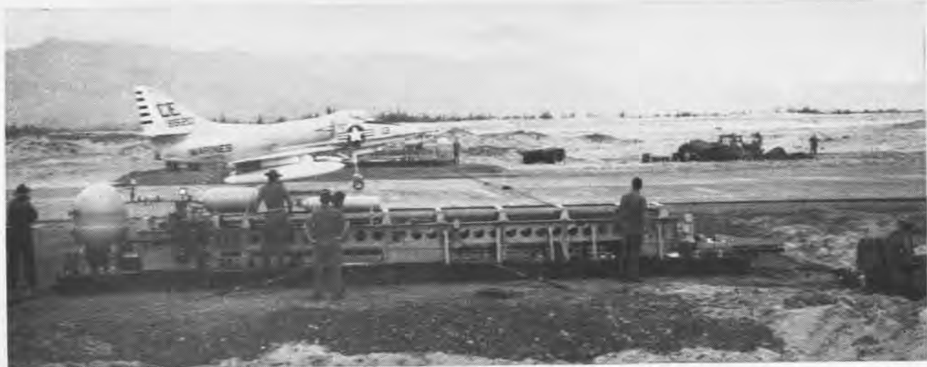
ITS TAILHOOK down to catch a MOREST cable, a Marine A-4 Skyhawk lands on the new expeditionary airfield at Chu Lai, Vietnam. The runway, still incomplete, was built of SATS panels by Seabees of MCB-10. Marines assigned to MABS-12 built support facilities.
