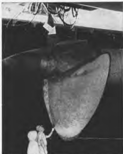
CORAL SEA C.O. inspects propeller after one of the blades broke off (see arrow).
