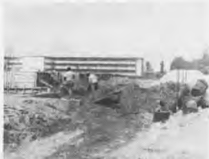
NEW CONSTRUCTION AT OCEANA
