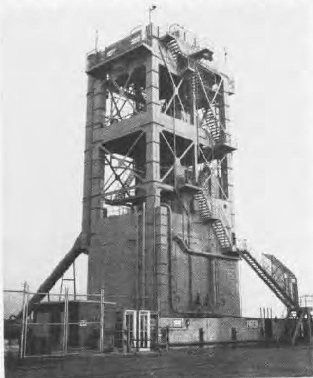
PROTOTYPE FUEL SYSTEM IS USED BY THE ABF SCHOOL
