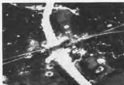
THI LONG railroad bridge was heavily damaged by A-4 Skyhawks flying from Ranger .
