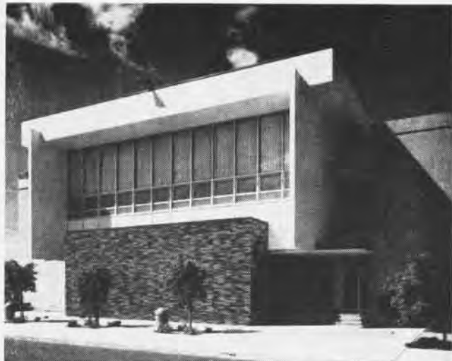
THIS NEW 40,000-square-foot building at the Pacific Fleet ASW School, San Diego, houses the complex 14A6A tactics trainer.
