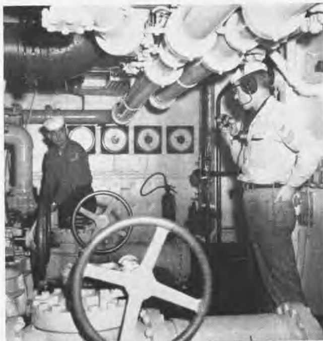
OPERATORS MAN AVGAS PUMP ROOM IN PROTOTYPE
