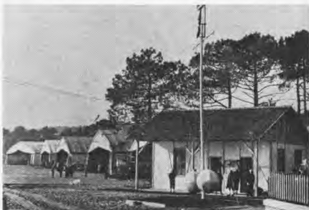
SIGNAL FACILITY AT MOUTCHIC, A TRAINING STATION IN FRANCE
