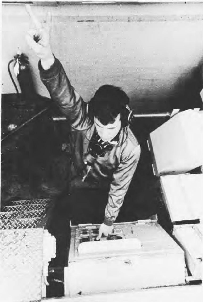
A Phantom moves onto the C-7 catapult site at NATC Patuxent River, opposite page. The boiler system for generating steam is under the catapult. BT2 Richard McMillan, left, prepares to light-off one of the destroyer-type boilers and bring it on the line. ABE3 Harold Maxwell, below, stands in a deck edge well with two fingers up, signifying the status of the launch is standby. After final clearance at this stage, launch is next.
