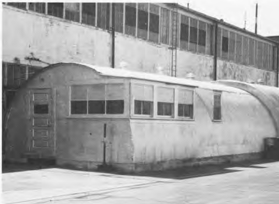
Camp Green, above, in July 1927, was headquarters for the Rhode Island State Militia and the landing field for Charles Lindbergh's barnstorming tour of the U.S. The Quonset hut, right, was designed by Quonset engineers after a suggestion by Adm. Ben Moreell, founder of the Seabees.
