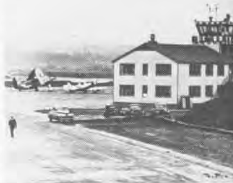
Photograph above is the Seaplane Base traffic control tower just after construction, November 3, 1945. Far right below is an oblique view of Ault Field as it appeared in 1944-45. One of today's squadron pilots, below right, inspects the bomb racks of his medium attack A-6 to make sure all is "go." Active NAS SAR team rushes a patient to an awaiting helicopter for medevac to a nearby hospital, right. This patient gave birth to twin girls en route to the hospital.
