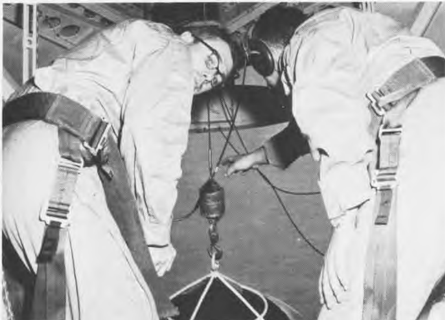
Crewmen winch salt water ballast aboard Snow Bird during the flight. This was done periodically to compensate for weight loss of consumed fuel.
