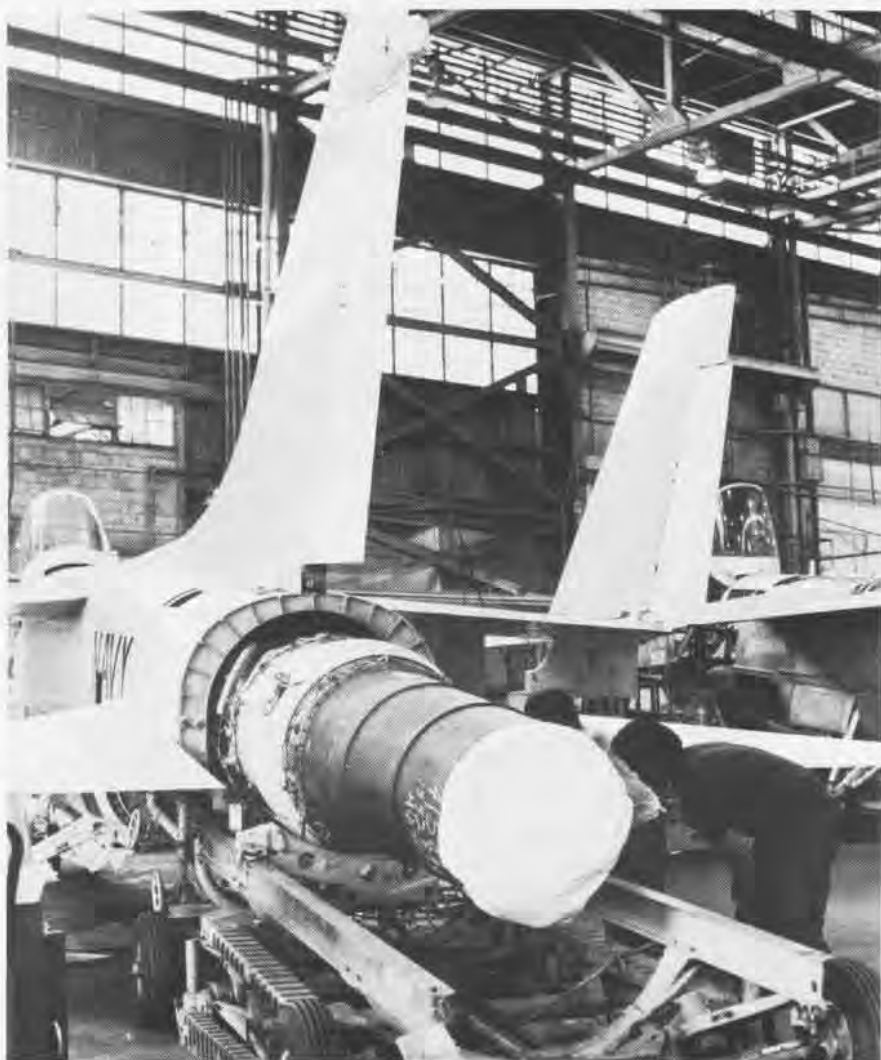
Above, A-7 Corsair II receives its engine during rework at NARF Jacksonville. Left, Tom Spruell of the nondestructive inspection shop examines X-rays of aircraft parts.
